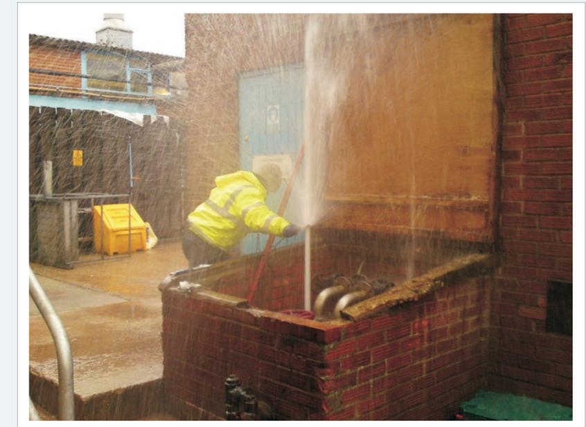
Photo 3: An example of Artesian conditions at well head. As well as being a waste of water uncontrolled conditions over time deplete the Aquifer and depress the local water level and therefore affect other users of the groundwater.
