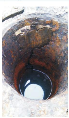
Photo 1: Deteriorating casing creates a pathway into the borehole
