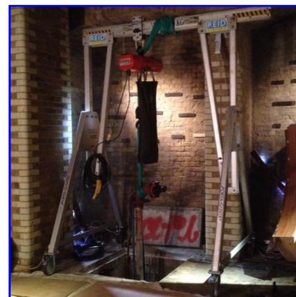
*A portable gantry set-up over a borehole located in a basement.*
