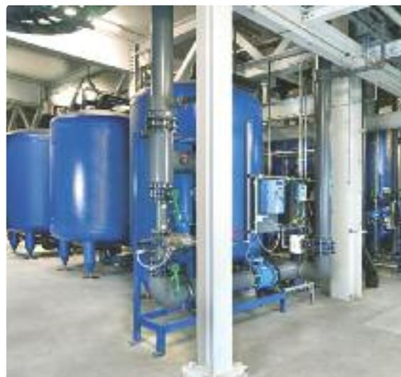
**A 200m<sup>3</sup>/hr water softening plant and blending unit with hardness monitoring in a modern Dutch brewery.**
