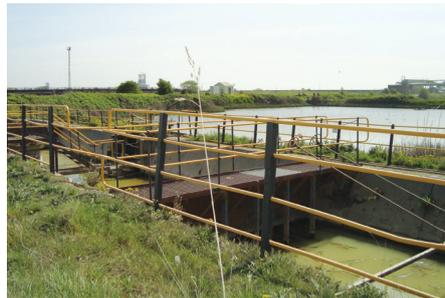
Assuming that the lagoon size is right, improved settlement can be achieved by using flocculants, but too often dosing is ineffective because of poor mixing when using blocks or liquid. It is therefore important to introduce flocculant in a turbulent flow regime to ensure mixing and then allow the flow to distribute fully across the lagoon to minimise flow velocity and maximise settlement.
